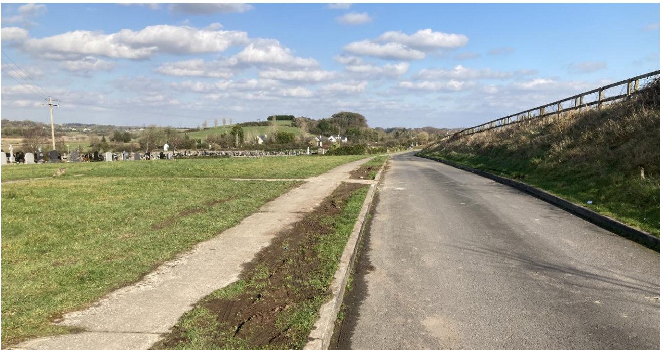
Figure 5 View of internal access road with subject to left and right
